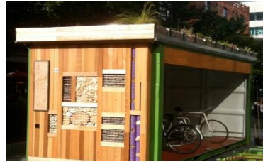
Green roof and timber cycle shelter.
