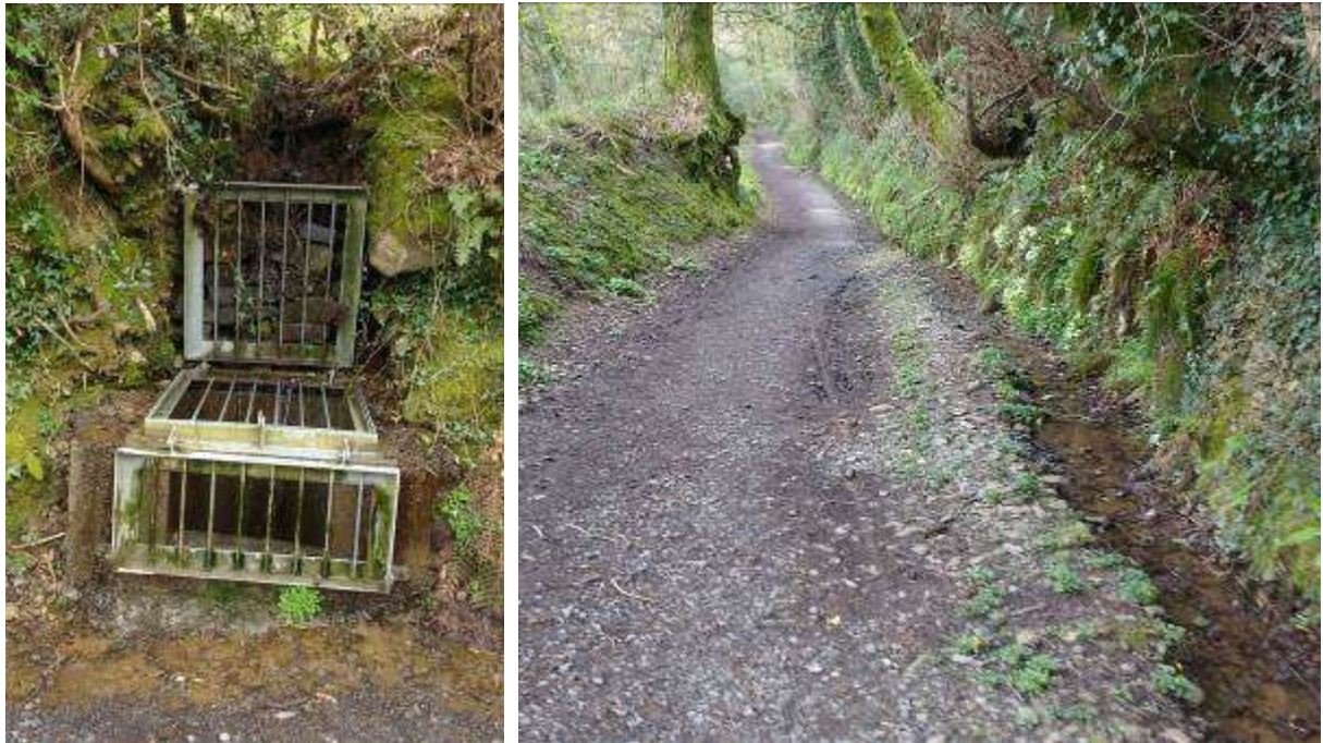
Photo's 3.5 and 3.6 – Existing drainage and overflow.
