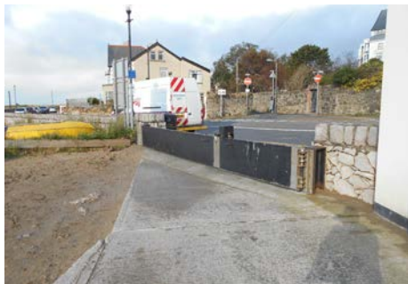
Existing flood gate in closed position at Marine Crescent and path near Deganwy Station that requires a new surface
