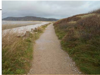
Cut back vegetation and widen path. Overlay with tarmac surface
