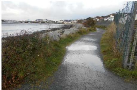
Existing dust path south of Deganwy Quays
