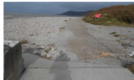
Existing path north of Deganwy Promenade that is exposed to some coastal erosion and vegetation encroachment on existing path edges
