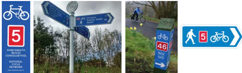
Examples of a repeater sign, directional signs, short robust posts and a shared pedestrian and cycle sign
