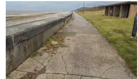
Existing flood gate in closed position at Deganwy Promenade and damaged surface at northern end of Promenade
