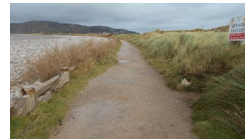
Existing path north of Deganwy Promenade that is exposed to some coastal erosion and vegetation encroachment on existing path edges
