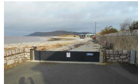
Existing flood gate in closed position at Deganwy Promenade and damaged surface at northern end of Promenade
