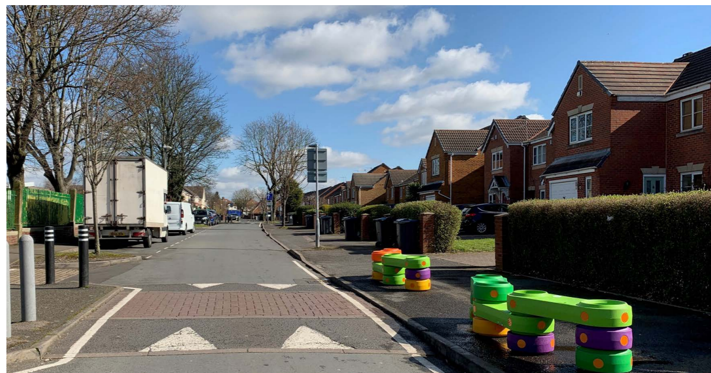
Fig 12. Trial to prevent pavement parking at the school in Pype Hayes. Image Credit: Sustrans
