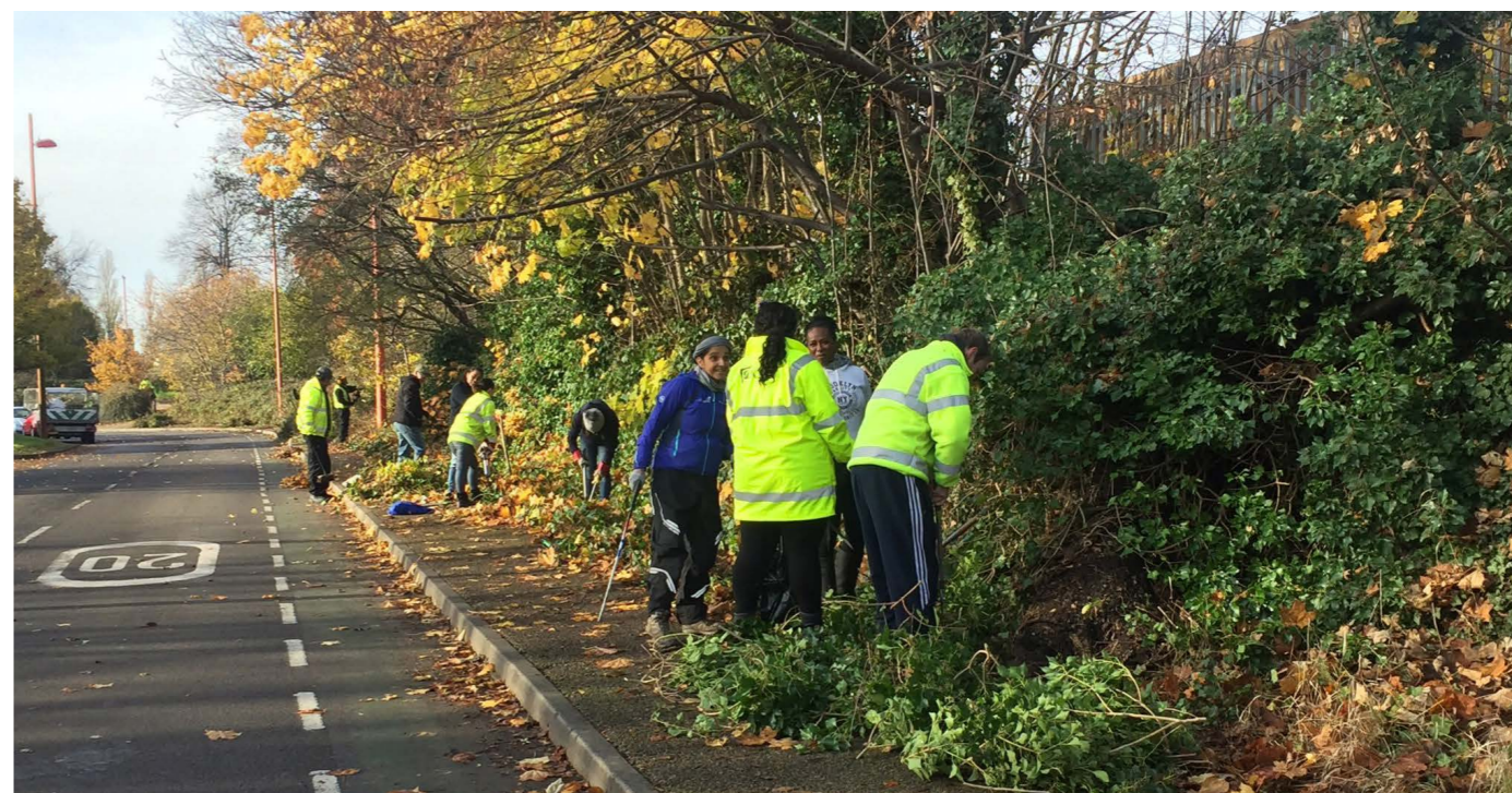
Fig 28. Clearing vegetation from pavements in Tyburn. Image Credit: Sustrans
