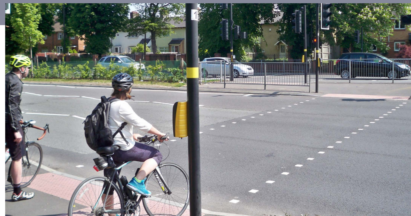
Fig 10. Combined pedestrian and cycle crossings Image Credit: Sustrans
