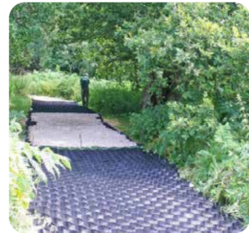
An above-ground no-dig construction method will be used to protect existing trees. Image source: Geosyn.co.uk
